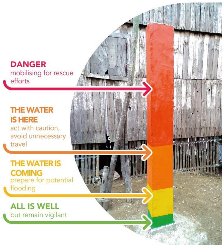
As soon as the masonry work is finished, the markings made by the people and the topographical data are transferred by the surveyor to each beacon. After that, the warning bands are defined in a participatory way and painted in green, yellow, orange and red colors.
