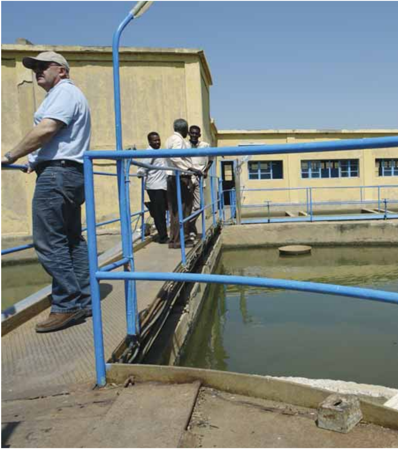
Photo: a water treatment facility in Gedaref, Sudan
